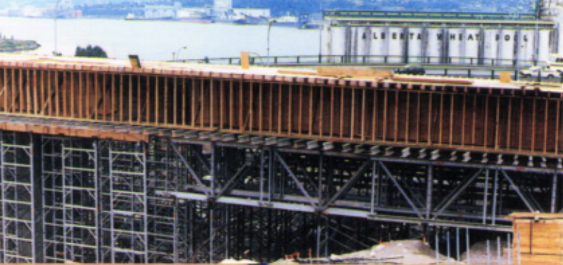
Pont Second Narrows, Vancouver, C.B.
